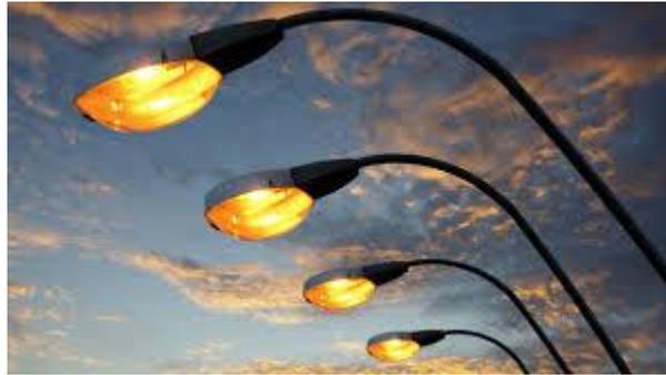
**2. Mercury Vapour Lamp:** A mercury vapour lamp is filled with mercury vapours (gas) instead of sodium and argon. Its working principle is identical to that of sodium vapour lamp. These lamps emit different coloured lights when different activators are added.
